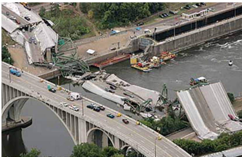
On 1 August 2007 the entire span of the I-35W Minneapolis bridge broke into sections and collapsed into the Mississippi River, resulting in 13 dead and 145 injured. In the eight years since, investment in infrastructure has collapsed, too.
