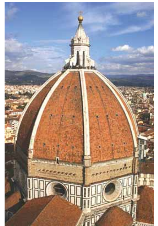
Filippo Brunelleschi discovered the universal principle of the catenary and used it to construct the dome of Santa Maria del Fiore, in Florence, which was completed in 1436.
