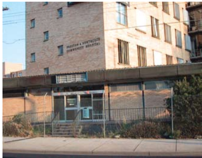
The Preston and Northcote Community Hospital (PANCH), a locally-run hospital, was taken over by Kennett's new health care networks, and shut down in 1998. The site was turned into student accommodation.
