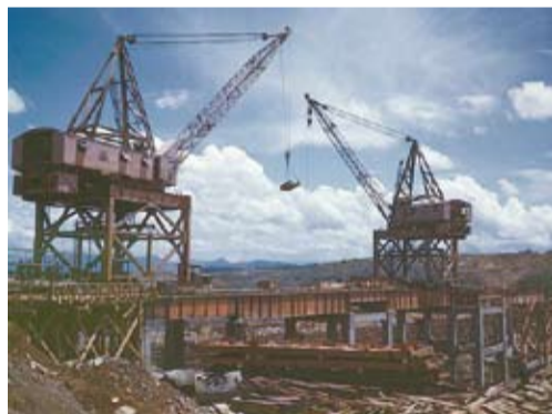
Construction of the Tennessee Valley Authority.
