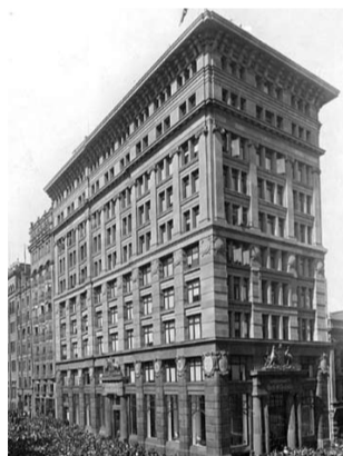
Commonwealth Bank headquarters, Martin Place, Sydney.
