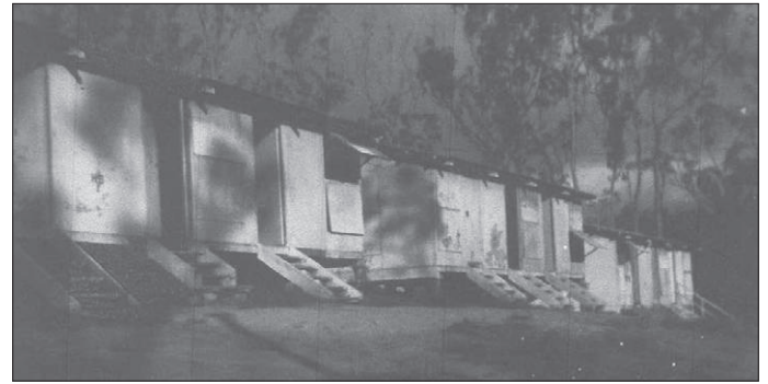
These prefabricated huts replaced the survey team’s original tents.
